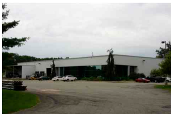
Our Role: Project Architect / Project Manager Architect of Record: Omega Design
